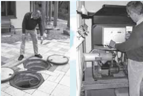
Paved area with shaft covers for the underground filter and cistern (left). Mechanical room with pressure boosting system and rainwater distributor to toilets, washing machine and irrigation taps (right).
