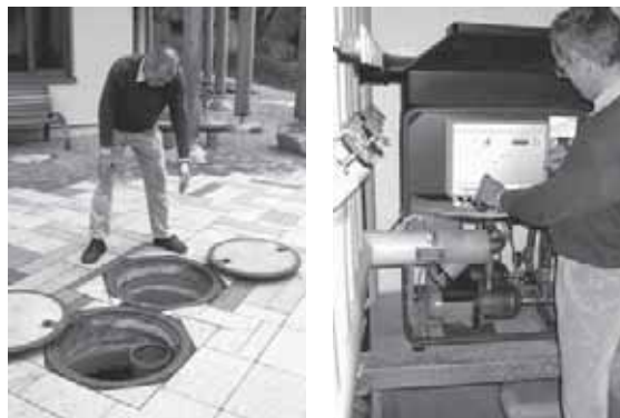
Fig. 1: Separate tapping points for wash water left drinking water, right cistern water
